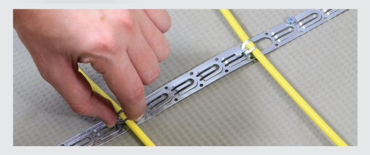
Thermoduo™ is a heavy duty 5.5mm underfloor heating system designed for use in concrete screeds and suspended timber floors.
